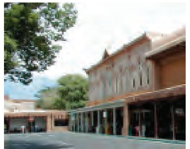
Santa Fe Plaza, east side. At right, the 1891 two-story Italianate Catron Block across from the Palace of the Governors, the oldest public building in America.
